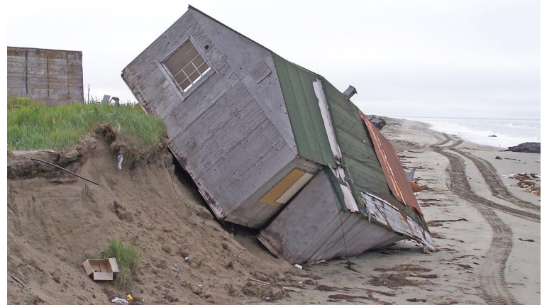
Eroding coastlines and melting permafrost damage facilities near Bering Landbridge National Preserve. NPS photo.
